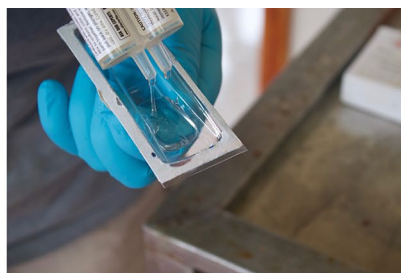
b Mixing the epoxy components
