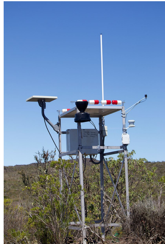
Fig. 3 Gateway relay station. The metal structure was assembled at the Galápagos National Park station to conduct final tests, prior to its deployment in the field
