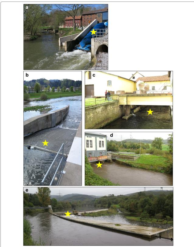
Fig. 1 Release sites of dead Atlantic salmon smolts and European silver eels. Release sites of dead Atlantic salmon smolts and European silver eels indicated by *yellow stars*: **a** in an Archimedes screw turbine in the Diemel, **b** on top of movable bulb turbine in the Kinzig, **c** in a tailrace of two Francis turbines in the Diemel, **d** in a tailrace in the Sieg and **e** in a spillway gate in the Sieg
